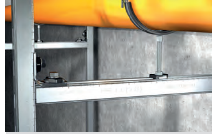
Pipe fixing on frame construction
