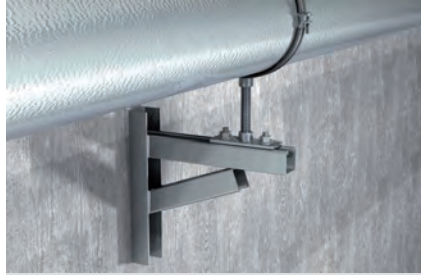
Upright pipe on cantilever arm
