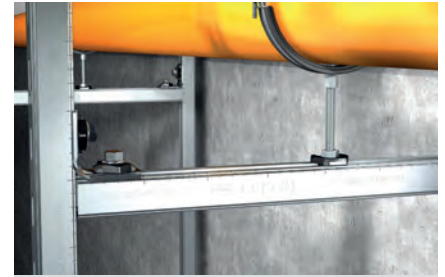
Pipe fixing on frame construction
