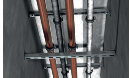
Pipe fixing in a corridor
