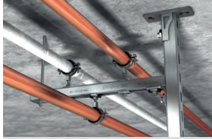
Cantilever construction with channel
