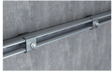
Channel installation at wall
