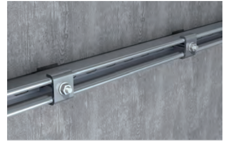
Channel installation at wall
