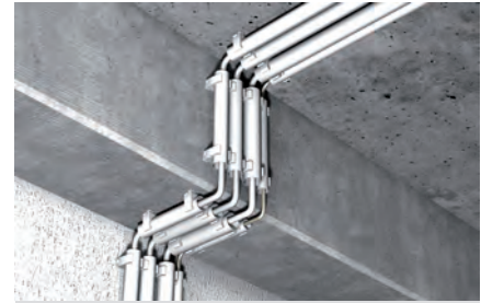
Fixing plastic insulating conduits
