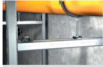
Pipe fixing on frame construction
