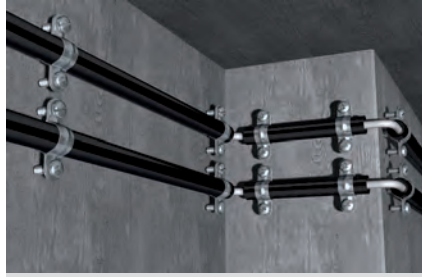
Fixing steel armoured conduits
